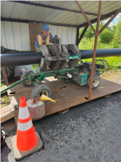
WATER DISTRICT #7 North Country Contractors hard at work!
